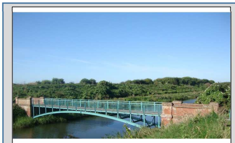
Seaview Bridge from North of the canal looking SW over Princes Parade. Houses will protrude over the bushes.
